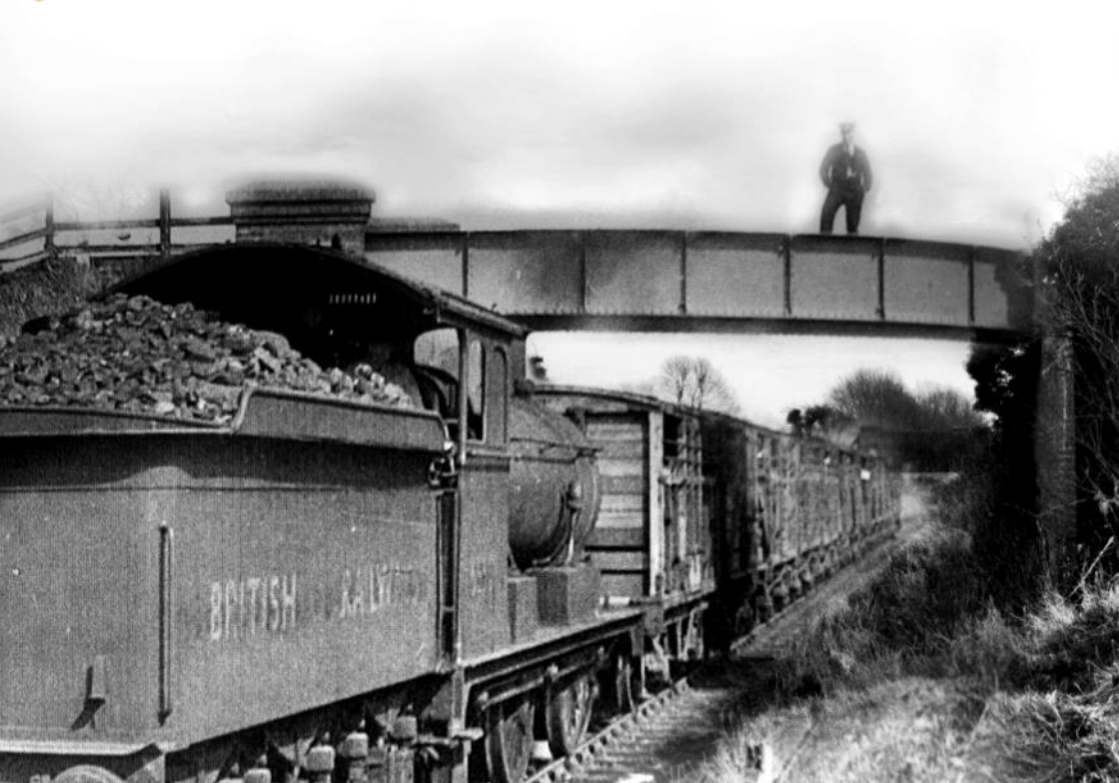
The bridge of the M&GN crossing the GER line near Themelthorpe, circa 1950. Image courtesy of Stuart McPherson.
